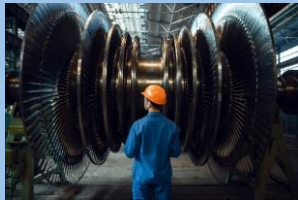
Electrical and Mechanical Service
